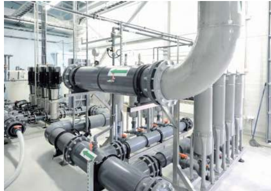
Municipal water supply
